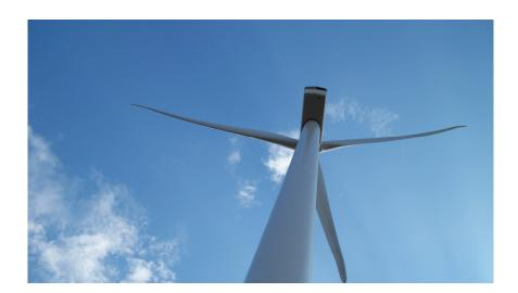
The nacelle with contents weighs about 70 tons (generator, gearbox, electrical cabinets, all equipment) and is the size of several pickup trucks. You would never guess the size when standing on the ground. Access to the nacelle is via a single straight ladder inside the tower, with two platforms on the way up. On a good day an agile and rested maintenance person can climb up in about 5 minutes, but 10 to 15 is more typical.
